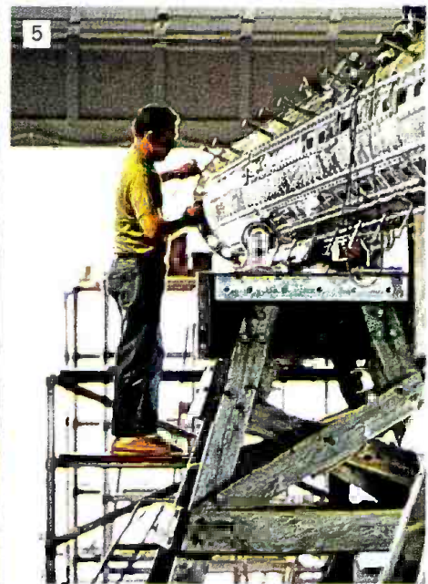
(5) Assembling one of the largest Pylon Antennas ever built. It will provide a base for a large Super Turnstile antenna in a stacked antenna arrangement.
