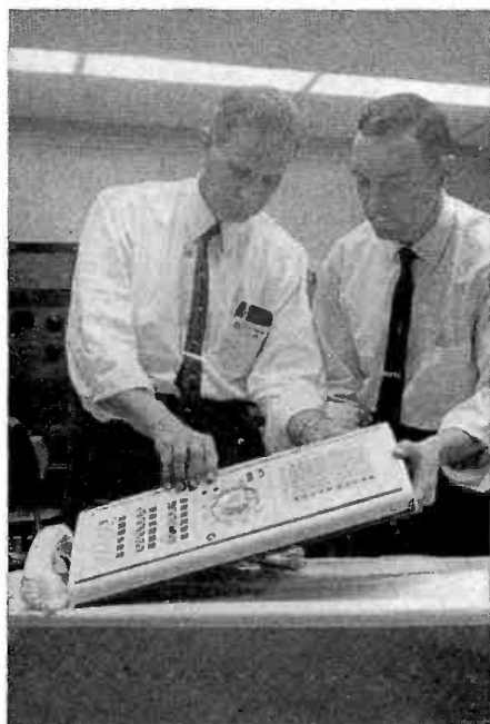
Bell Telephone Laboratories and Western Electric engineers worked together in perfecting this new cordless switchboard console which gives modern push-button convenience in a compact shape. A new console is examined by W.E. Planning Engineer Harold Haynes (right) and B.T.L. Design Engineer Robert Wirsching at Western Electric's Indianapolis Works.
