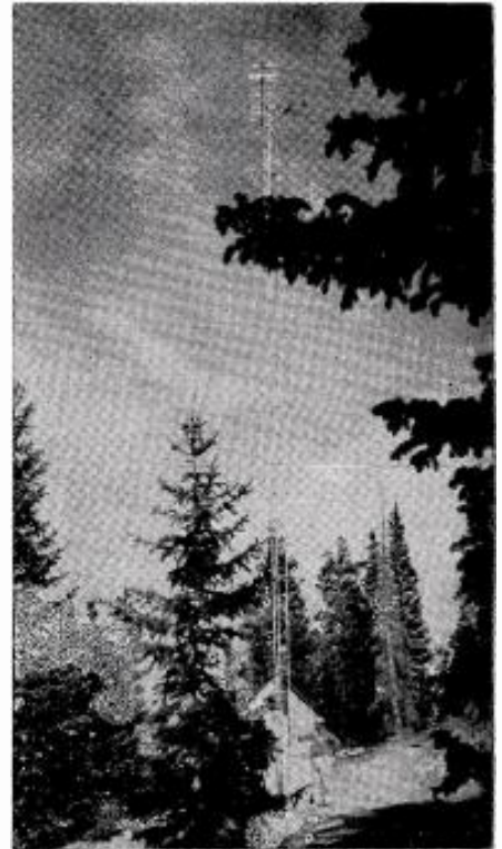
Among the evergreens 10,500 feet up Round Top Mountain sits this tiny shed housing a 1 w vhf translator that provides tv service from KREX-TV Grand Junction, Colo., to canyon-isolated Lake City, 100 miles away. (See Lake City panorama on page 69.)
