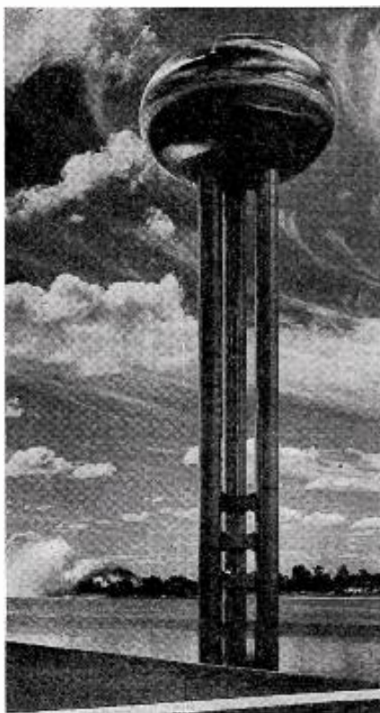
This stainless steel water tower is a landmark of the General Motors technical center near Detroit.
