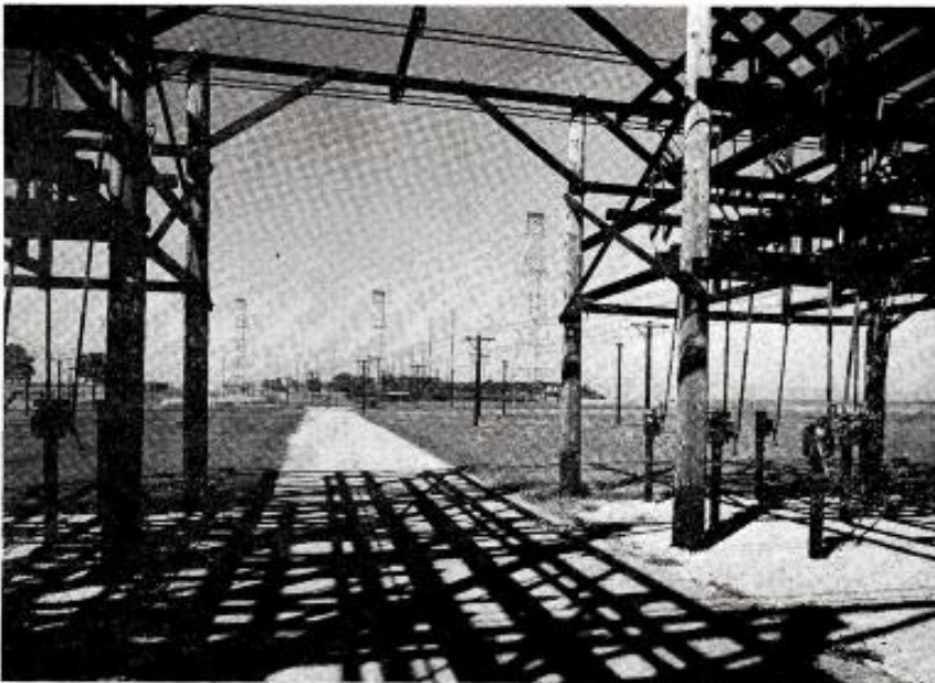
Shadows of some of the 20-foot poles in a forest of 232 switches which can be manually operated from the ground to connect any of the six transmitters with any of the 22 antennas of the VOA facilities at WLWO, are maintained and operated by Crosley Broadcasting Corporation as a relay base for broadcasts.
