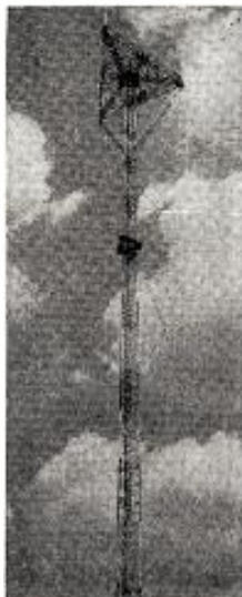
Super strong legs of USS "T-1" Steel support the tremendous weight of the tower. Their smaller size reduces wind resistance.
