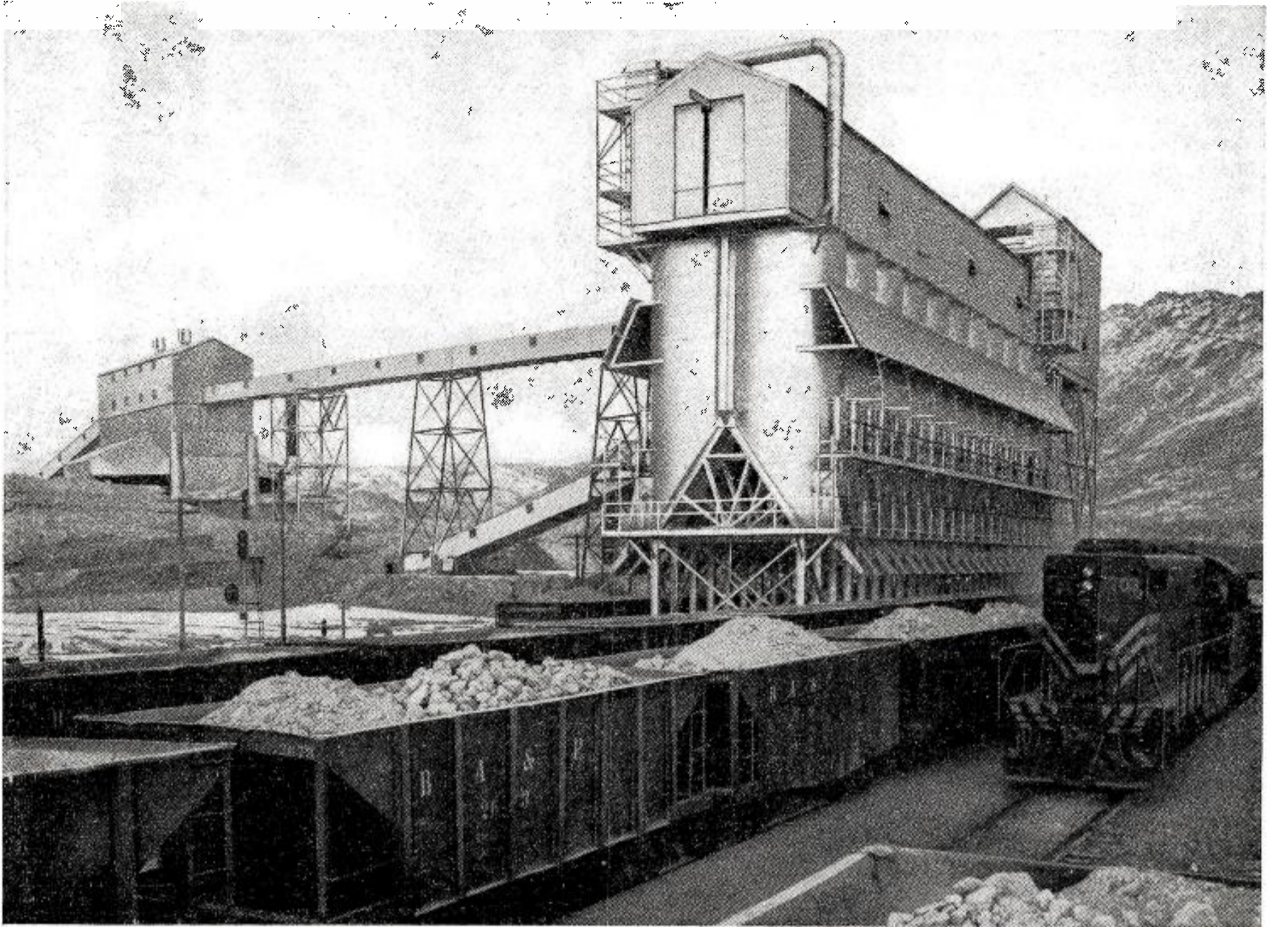
Fast, efficient handling is essential to the economic processing of low-grade ore. This new conveyor hauls ore out of the Berkeley Pit at the rate of 33 tons a minute.
