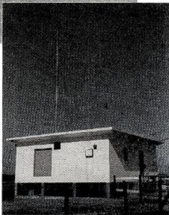
Compact Installation—at KLIF 50 KW transmitter site.
