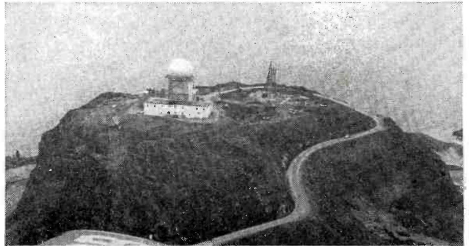
DEW LINE of radar stations, built by W.E. for the Air Force in 32 months, is now being extended across the Aleutians. Hundreds of Bell System people bucked the Arctic to help build it.
