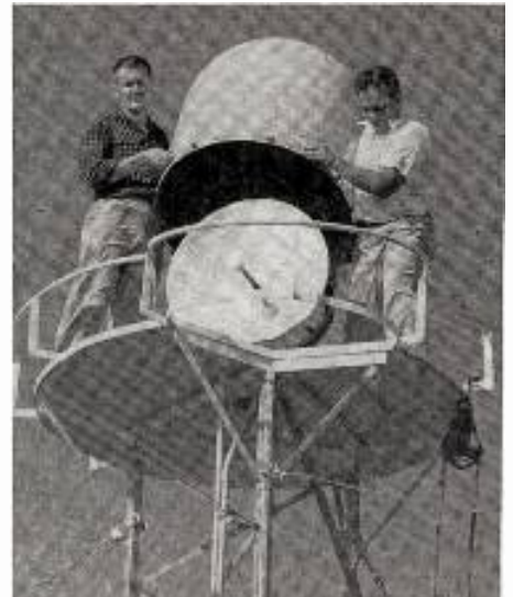
Engineer Eldon Kagano (1) and assistant engineer Verne LaBrayere, who installed the set, boost the "blister" to show "dish" sending-receiving antennas. These are mounted atop a 50-foot tower.
