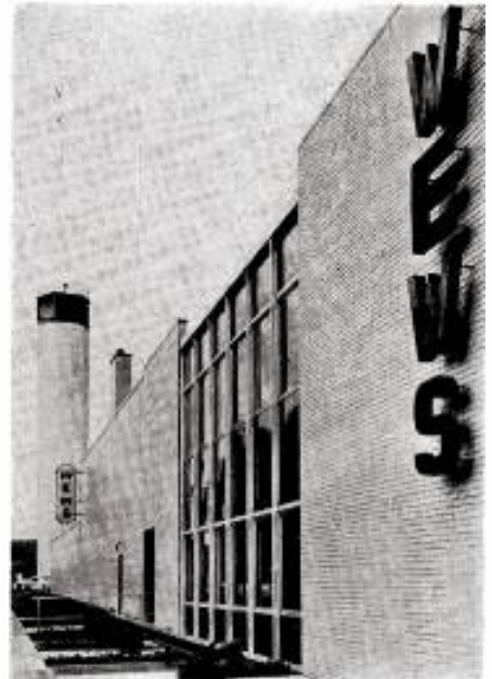
RIISING above the new offices and studio of WEWS (TV) Cleveland is the unusual concrete silo microwave tower erected by the Marietta Concrete Corp., Marietta, Ohio. The 100-foot silo tower houses the parabolic antennas used to direct the broadcasting signal to the station's outlying transmitter in nearby Parma, Ohio. Unlike the conventional open-work microwave towers, according to a report from Marietta Concrete, the parabolic antennas in the WEWS tower are enclosed behind the plexiglass windows which eliminate outside weather interference, particularly picture bounce caused by high winds.
