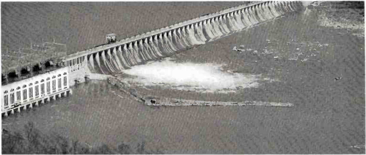
This power dam was built on the Susquehanna River near the Pennsylvania-Maryland border by the local independent electric light and power company at no cost to taxpayers.
