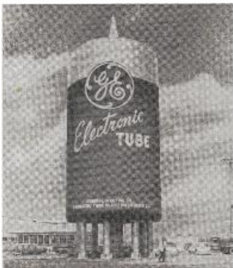
THIS 80-ft., 200,000 gallon water tower has been constructed at the site of a new General Electric tube factory now under construction in Owensboro, Ky. The tower is modeled after 6BK7-A, a vhf tube used in tv sets. Its real-life counterpart is only two inches high.
