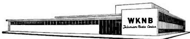
STUDIOS AND OFFICES • WEST HARTFORD, CONN.
