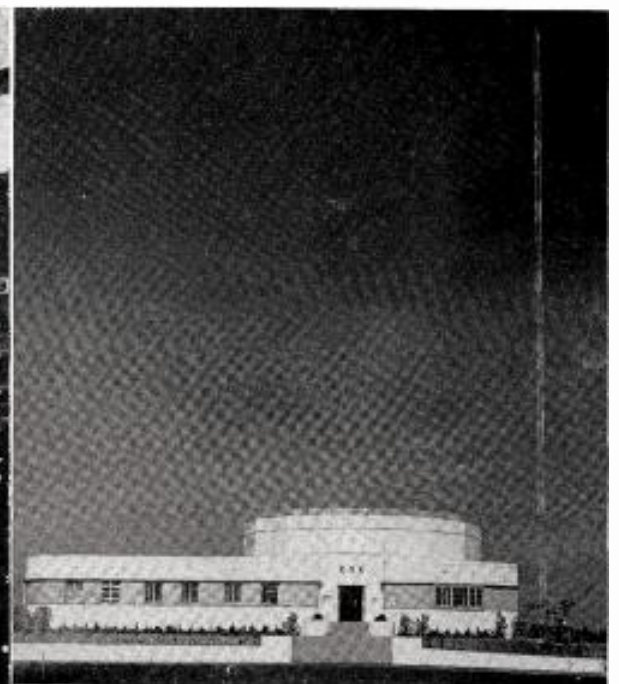
NOW 35 years old, KNX signals emanate from this modern transmitter building at Torrance, Calif.
