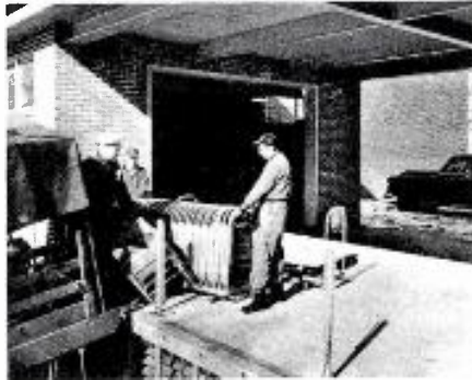
Loading ramp adjoins TV studios... permits truck unloading at bed level on one side; driving of autos from 100-car parking lot on other side.
