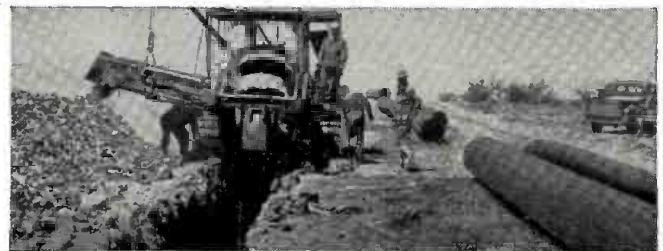
Goodbye Gas Shortage. For years now, gas companies have been rapidly laying new pipelines to ease the gas shortage. The job has been made easier with this giant trenching machine made from USS MAN-TEN Steel. MAN-TEN has such high strength that the machine can be made stronger and lighter than with carbon steel.
