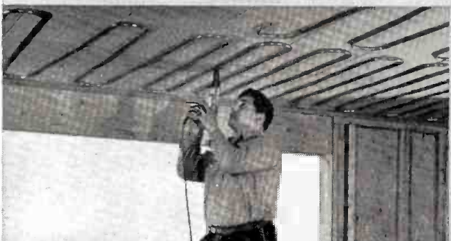
Brass Mills. New pre-formed copper tube grids for radiant panel heating come from The American Brass Co., an Anaconda subsidiary.
