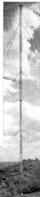
Slender 275-foot insulated tower for AM radio
