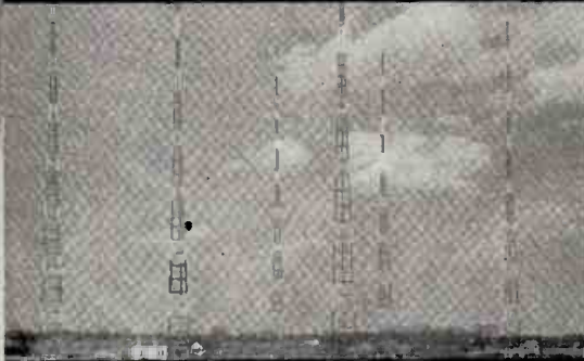
WFMJ-FM Truscon Self-Supporting Directional Towers, 400 Feet Tall
