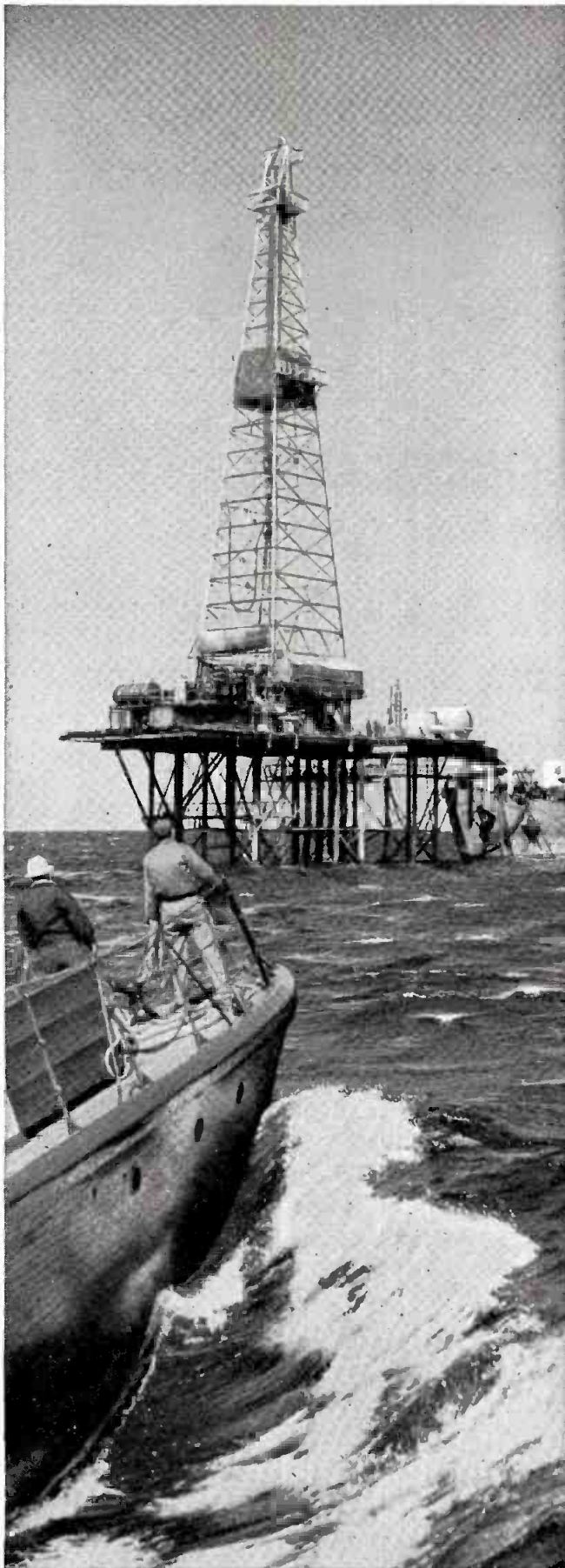
OFF LOUISIANA COAST , supply boat plows through choppy seas to offshore rig. Because of difficulties of exploring and drilling at sea, of bad weather, and of communication and transport problems, cost of getting oil from under the Gulf is 2½ to 3 times that of oil produced ashore. Yet competition is so great, oilmen will drill offshore more than a well a week this year.
