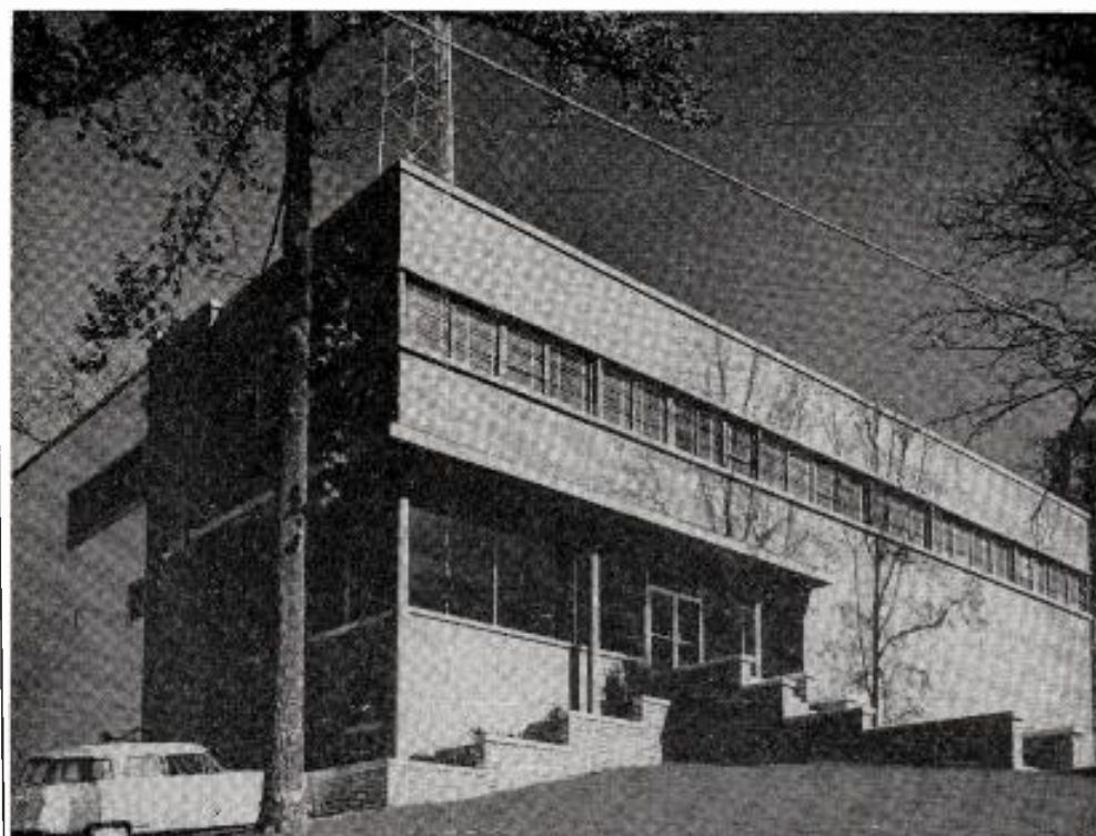
WLWA (TV) Atlanta's new studios contain 36,000 square feet of floor space, including 50 offices and two large television studios, one seating 300 people.
