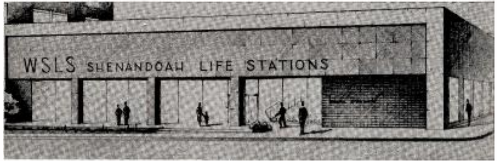
WSLS-AM-FM-TV Roanoke's half-million-dollar radio-tv center, expected to be complete in September 1954, will offer passersby a view of a tv studio where programs are in progress. Six windows (at right) will display products advertised on WSLS radio and tv programs and photographs of stars of the respective shows.
