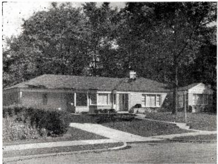
NEW ELECTRIC HOMES. This home for electric living was part of an exhibit co-sponsored by Indianapolis Power and Light Company. It features planned kitchen, improved lighting, year-round temperature control.
