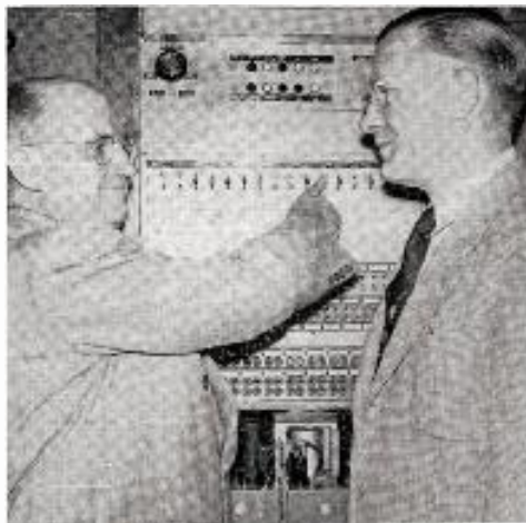
CONELRAD panel is discussed by KFI Los Angeles' co-chief engineers H. L. Blatterman (l) and Curtis Mason, who are responsible for its development from original specifications by the FCC. KFI held open house during the NARTB convention to explain how the installation functions.
