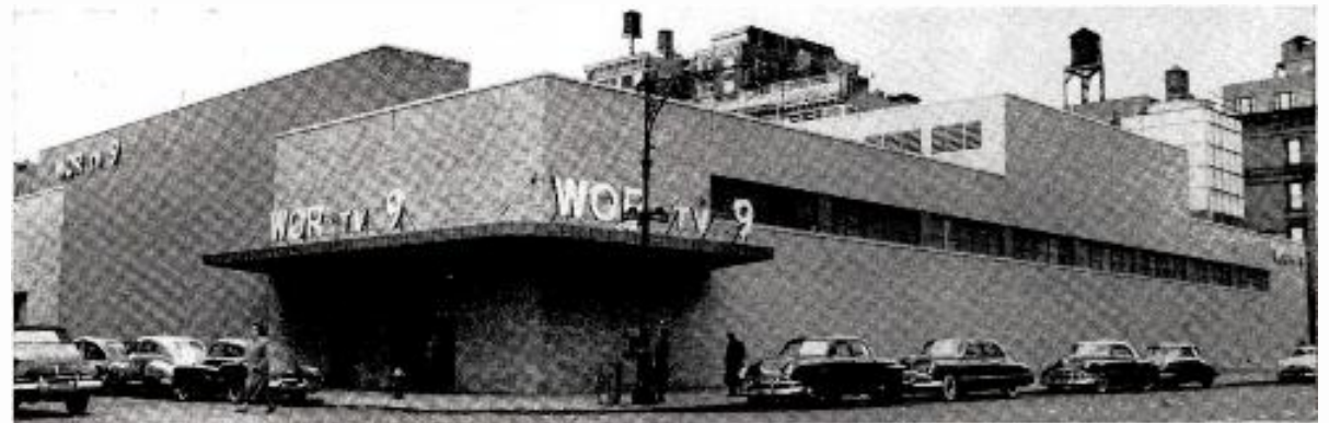
EXTERIOR view of WOR-TV New York's new Television Square which was formally opened Wednesday. The structure, at 67th St. and Columbus Ave., was erected and equipped at a cost of $3 million [B*T, Jan. 7]. It
