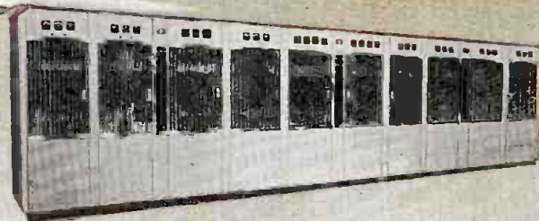
20 kw, for VHF Type TT-20BL/H (All Air-Cooled)
