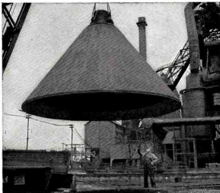
39 DAYS: This is the "bell" which caps a blast furnace. One steel company tore down an old blast furnace and replaced it with new one in one month and nine days.
