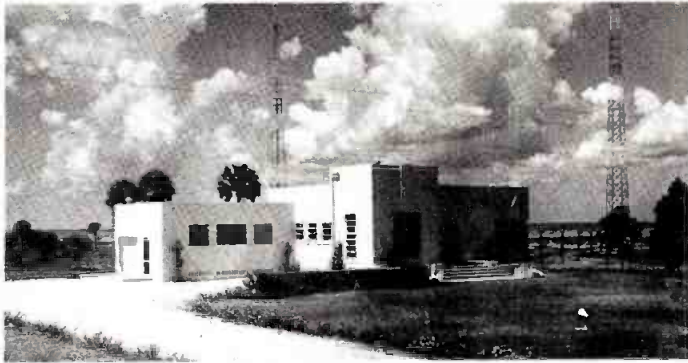
Modern Transmitter House
