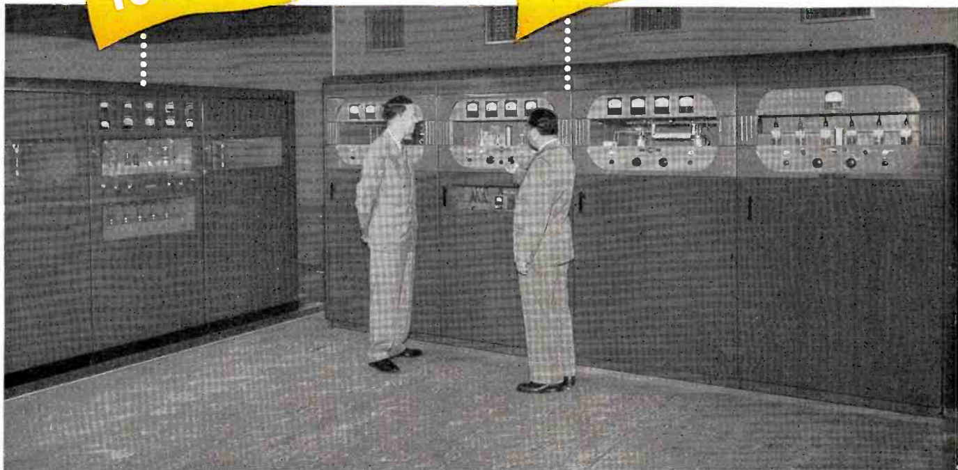
John Wildermuth, Chief Engineer, WADC (left), and his assistant, Larry Hennigan, with the new 21B 5 kw transmitter. The 21A, installed eight years ago, can be seen at the left.
