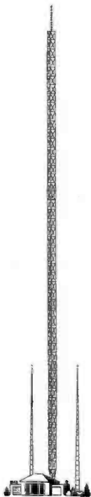
THE WORLD'S TALLEST TELEVISION ANTENNA . . . Built on top of the WKY-AM radio tower . . . 966 feet above the ground.
