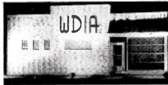
Sixth station to take the air in Memphis, WDIA, is housed in this modern structure.
