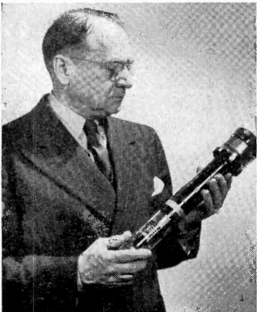
Dr. Zworykin with the Image Orthicon tube.
