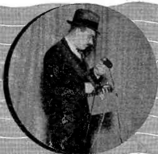
4. PORTABLE EQUIPMENT — This is the RCA OP-6 portable pickup equipment. A companion unit, the OP-7, provides a four-position, high-level mixing system also suitable for outside use.
