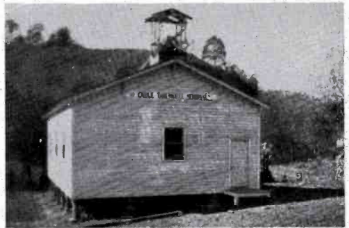
PREVIOUSLY ABANDONED, THIS ATHOL, KY. CHURCH now provides comfort for its mountinside area.
