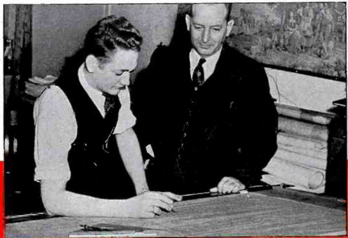
J. W. McDONALD (right), Assistant Technical Supervisor, discusses with Engineer Howard Laped a construction drawing of development work on Crosley's new 50,000 watt international short wave transmitter, WLW0, created in its entirety by WLW engineers.
