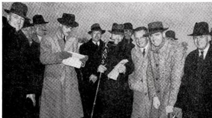
42D & BROADWAY, Wichita, Kan., is the locale for this picture of the groundbreaking ceremonies for the new transmitting plant of KFBI, which is to move from Abilene to Wichita early in February, 1940. Smiling in the mud during the first rain in several weeks, H. K. Lindsley, president of Farmers & Bankers Life Insurance Co., Wichita, owners of the station, and Herb Hollister, recently named vice-president and general manager of KFBI, put their feet to the spade for the first shovelful of excavation. Others in the group include J. Ward Gates, president of the Wichita Chamber of Commerce; Jack Todd, manager of KANS, at the microphone; K. V. Pyle, KFBI technical director; Mayor Frank Coleman, and Alfred MacDonald, city manager. KANS, using its mobile unit, scored a first by carrying the initial broadcast from the new KFBI site.
