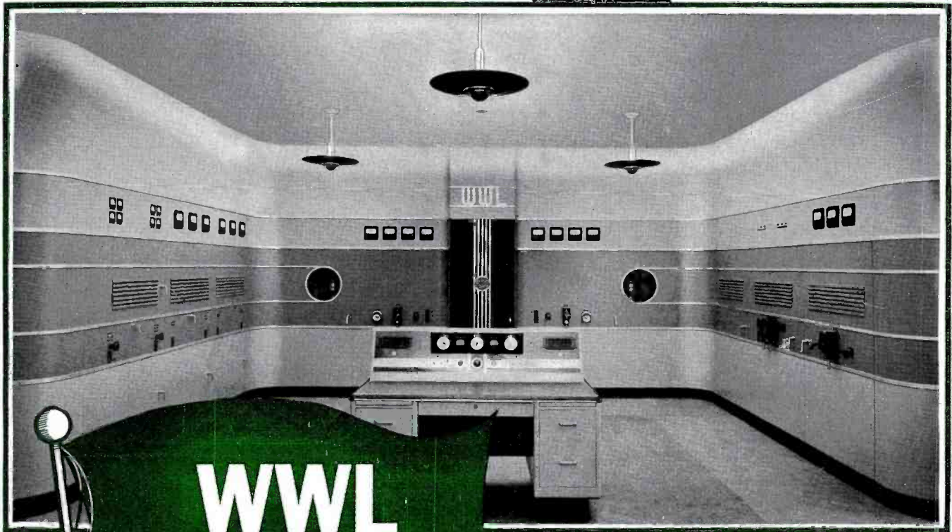
New U-shaped RCA 50 kilowatt High Fidelity transmitter just installed at WWL. It is Model 50-D.
