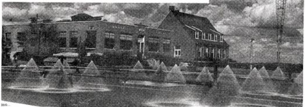
WLW transmitter plant at Mason, O. The spray pond in the foreground pumps a million gallons daily. The 500,000-watt transmitter building is at left, with operator's dormitory in center, 830-foot radiator, in rear.
