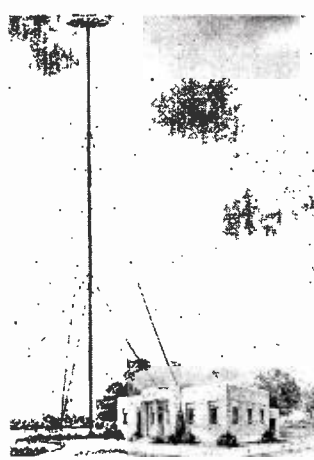
NEW WRC—Here is the new transmitter building of WRC, in suburban Washington, to be dedicated in latter March with its new RCA transmitter and 400-foot Truscon radiator.
