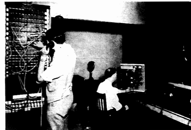
PATCHBOARD AND CONTROL ROOM—Fifty-four pickup points on the Century of Progress Exposition grounds are controlled from this point, off Studio H, and from here there are also lines to seven Chicago stations and to the two networks.
