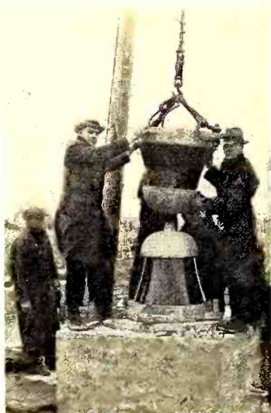
Base of 500 kw. WLW Mast
