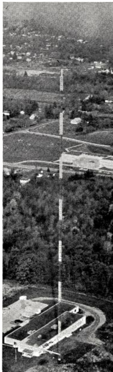
(WNYP-TV Tower installation at Jamestown, N.Y.)
