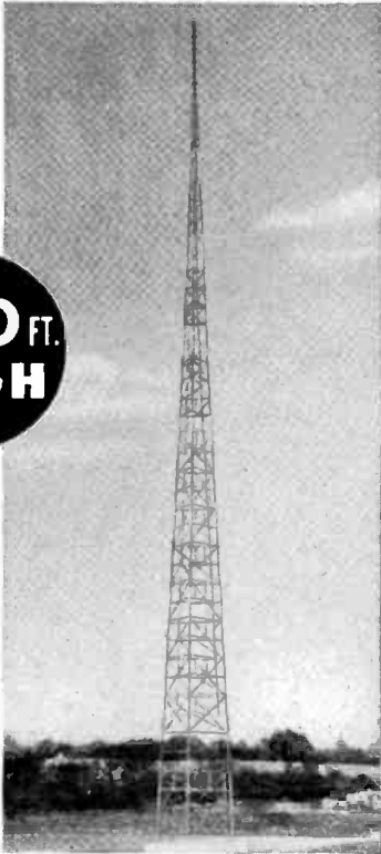
Above: Truscon Type H-30 Self-Supporting Steel Radio Tower climbs 500 feet high with an 8-bay Western Electric FM antenna for WPIC, Sharon, Pa. Overall height is 550 ft.
