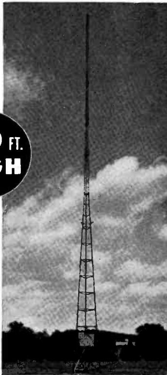
Above: 5000-watt WMAK, Nashville, Tenn., uses five Truscon Type A Self-Supporting towers, each 210 ft. high.
