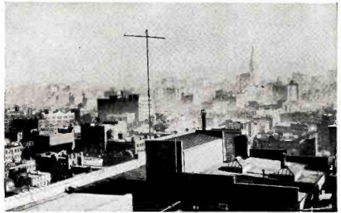
WEAF Antenna—1922. 463 West Street, New York City
