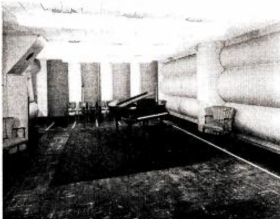
Studios equipped with Paly-cylindrical Wall sound treatment
