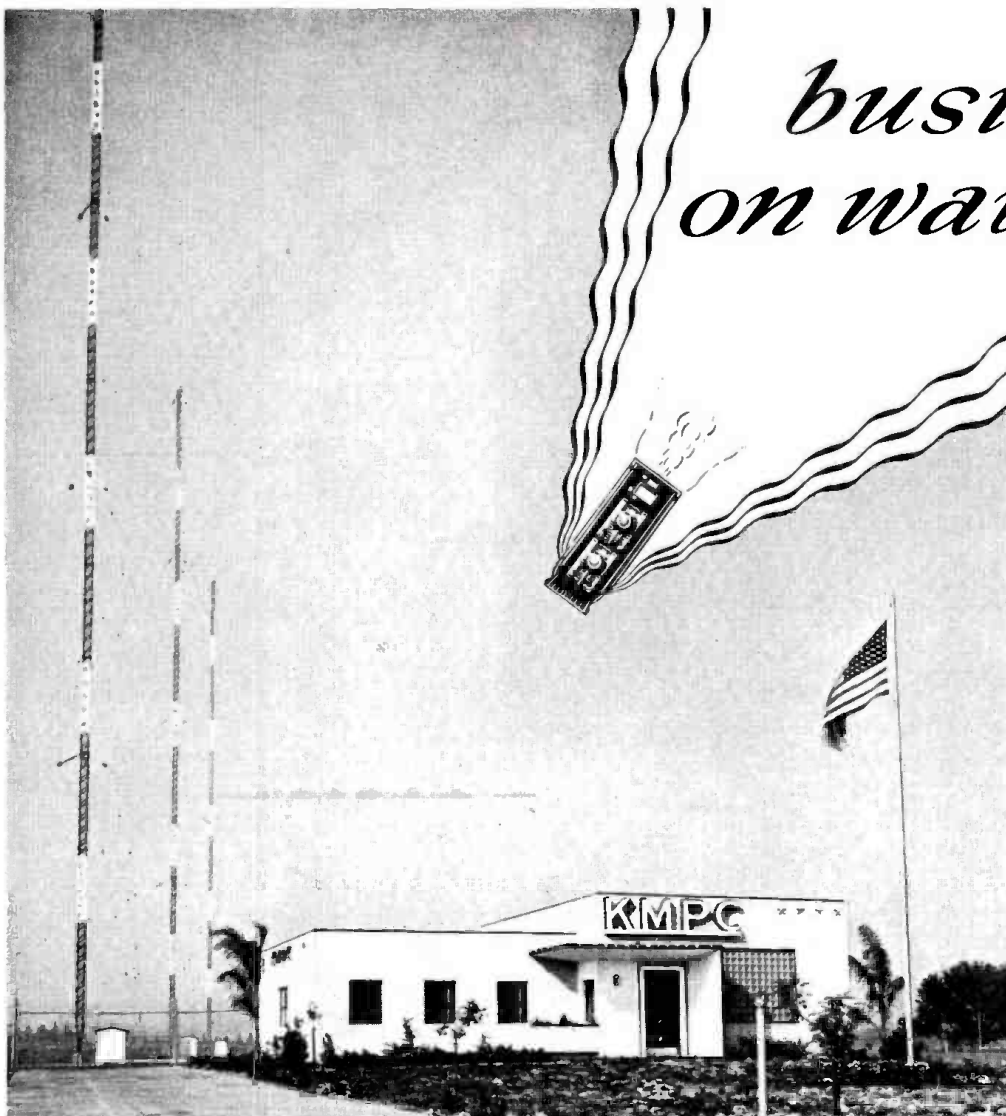
Illustration shows 3—300 foot Galvanized guyed Lehigh Vertical Radiators of Radio Station KMPC, Beverly Hills, California.
