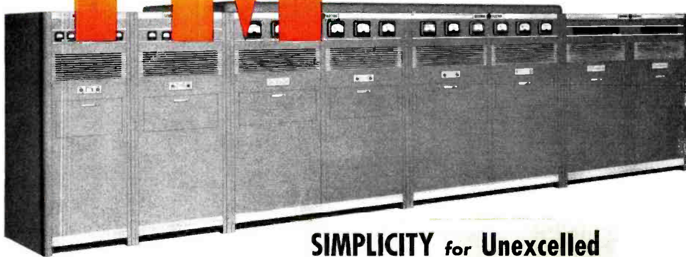
G.E.'s 50-kw FM transmitter takes only 101.8 sq ft of floor space for all equipment including water-cooling; uses the new high-frequency GL-880's in the final amplifier.
