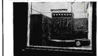
● All broadcasting equipment is of the most advanced type and expertly engineered.
