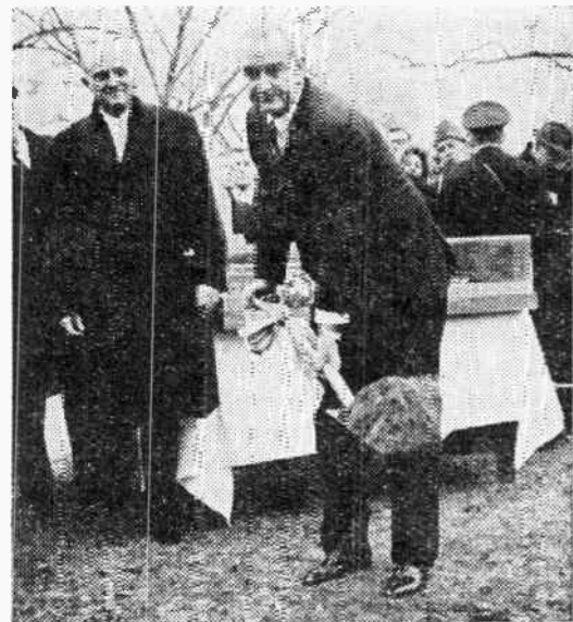
President Johnson breaks ground for the John F. Kennedy Center for the Performing Arts, with Roger L. Stevens, chairman of the Center's board of trustees, looking on.
