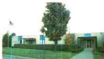
New Martin Facility
