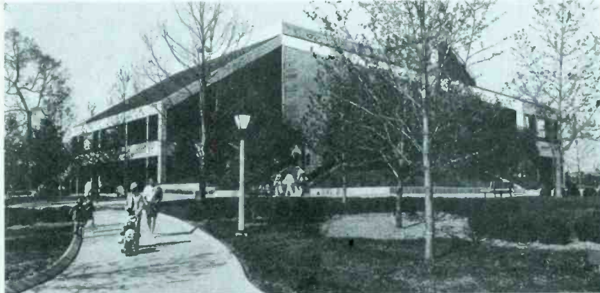
NEW OLE GRAND OPRY — Since its opening on March 16, 1974, the $15 million Opry House theatre and television production facility has been drawing the biggest names in entertainment to Opryland in Nashville for live stage concerts and network and syndicated television shows. Fifty-two weekends a year, the Opry House is the home of the Grand Ole Opry, the world's longest running live radio show which will celebrate its 53rd anniversary this fall.
