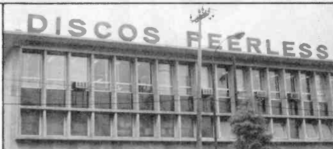
A section of the mammoth facilities on busy Avenida Mariano Escobedo.
