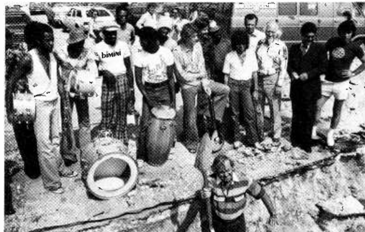
DIGGING FOR GOLD —Mack Emerman, president of Criteria Recording Studios in Miami, grabs a shovel and begins digging in at recent groundbreaking party for Criteria's fourth 24-track studio. Members of T-Connection, Funk Machine and Wishbone Ash took time off from sessions to look on as did Henry Stone of TK Productions (third from right).
